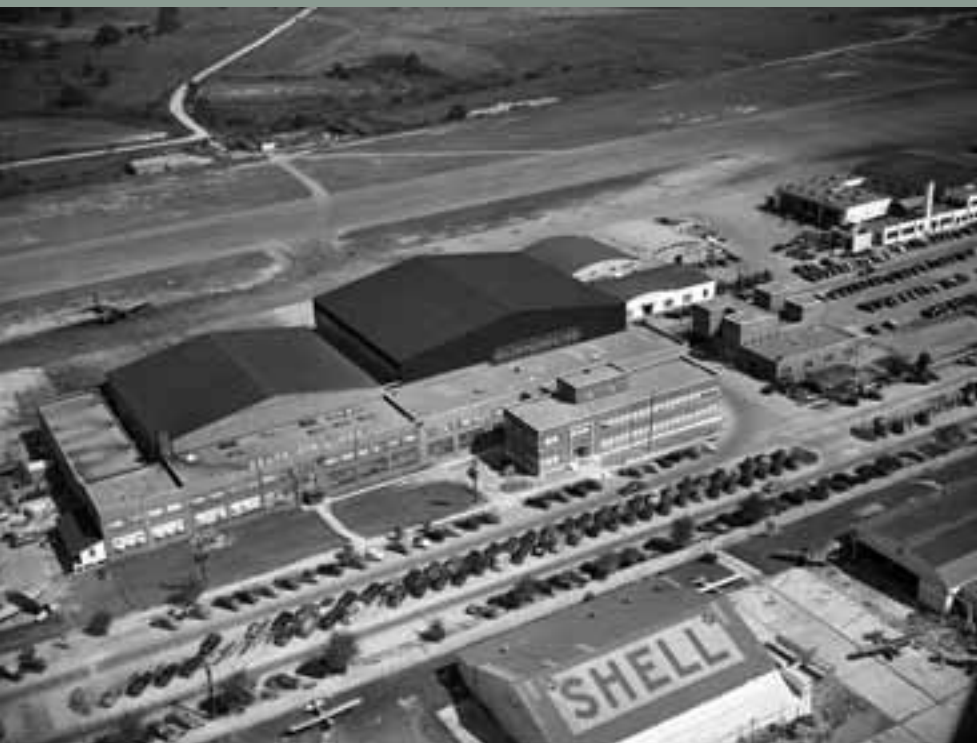
Delta's headquarters more than doubled in size in 1947, with a second larger aircraft hangar, with attached office and support facilities, and a new executive building in front.
