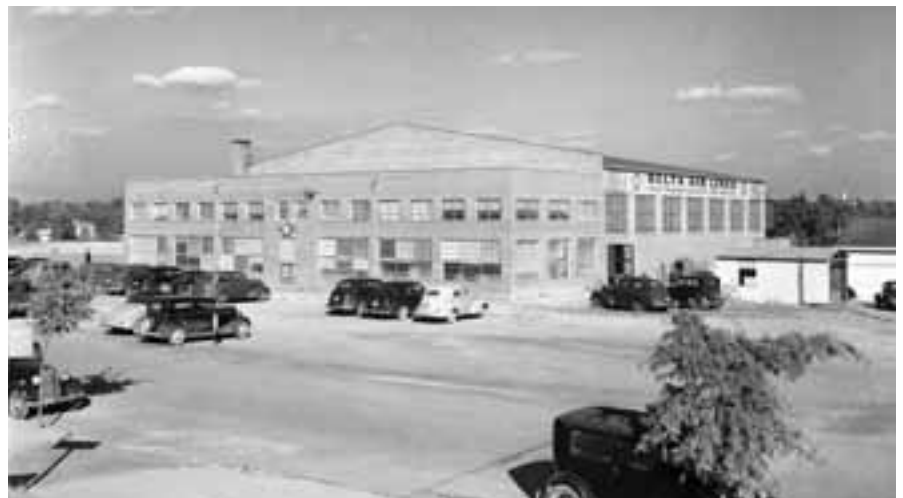
Delta’s original 1941 headquarters in Atlanta. The aircraft maintenance hangar—the largest one in the Southeast—and attached office building cost $150,000 to build.
