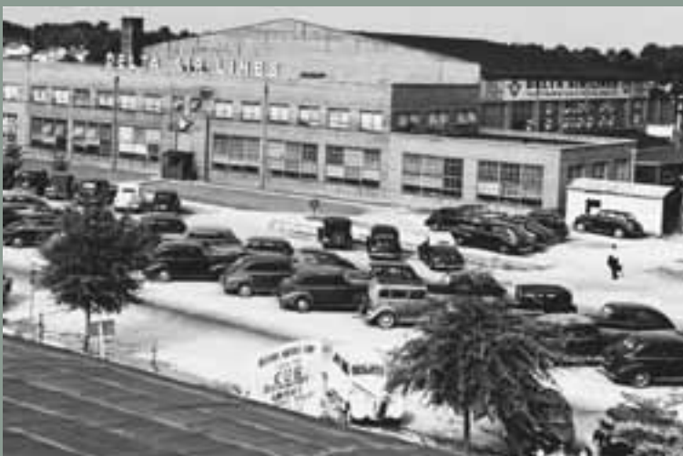
The original 1941 hangar and General Office Building, now with wings added in 1942–43. The one-story annex at right held the aircraft engine overhaul, accessory, and machine shops.
